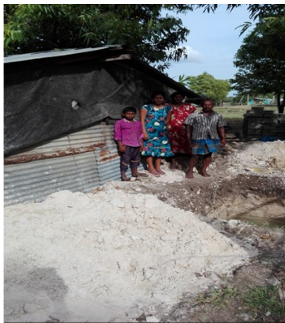
Resettlement of displaced people of Sampoor: Providing Toilets to Returning Families, Program initiated by Assist Resettlement & Renaissance, 15 of 25 Toilets supported by IMHO
