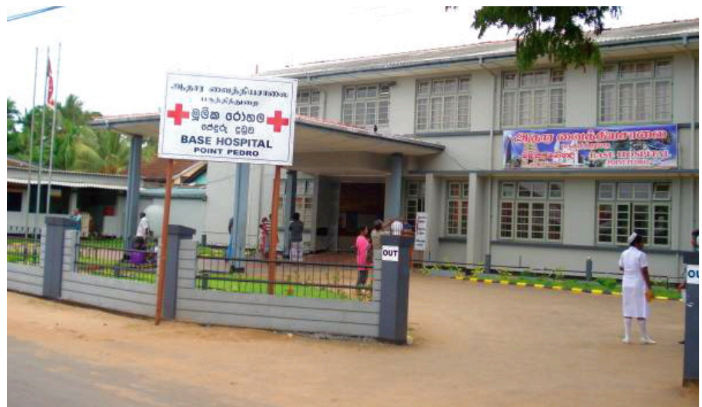
The newly renovated Point Pedro Base Hospital in Jaffna.
