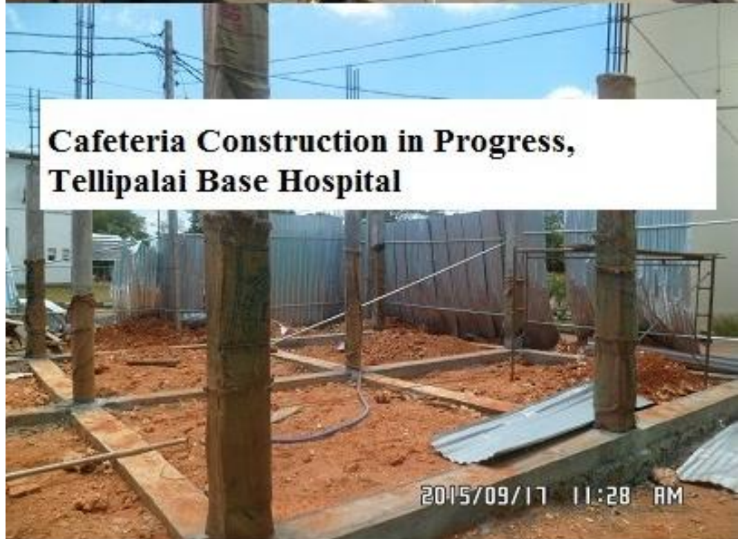
Cafeteria Construction in Progress, Tellipalai Base Hospital
