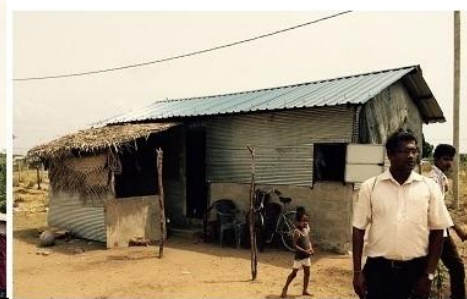
Sampoor Recently Built Housing- Additional Houses to be funded by IMHO
